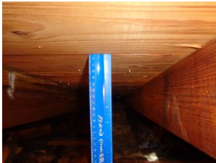
Garage, Basement & Attic Attic
