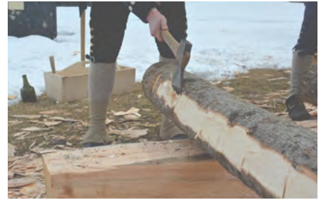
Provincial soldiers snap a line and carefully cut with their axes to hew round logs into useable square beams.
