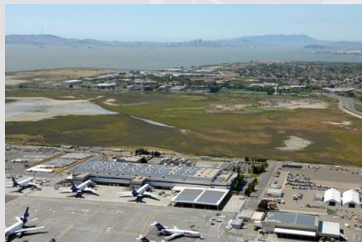
0.9 MW FedEX Building, Oakland, CA
