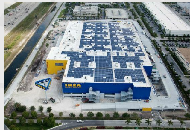
178,000 Sqft IKEA Solar Rooftop
