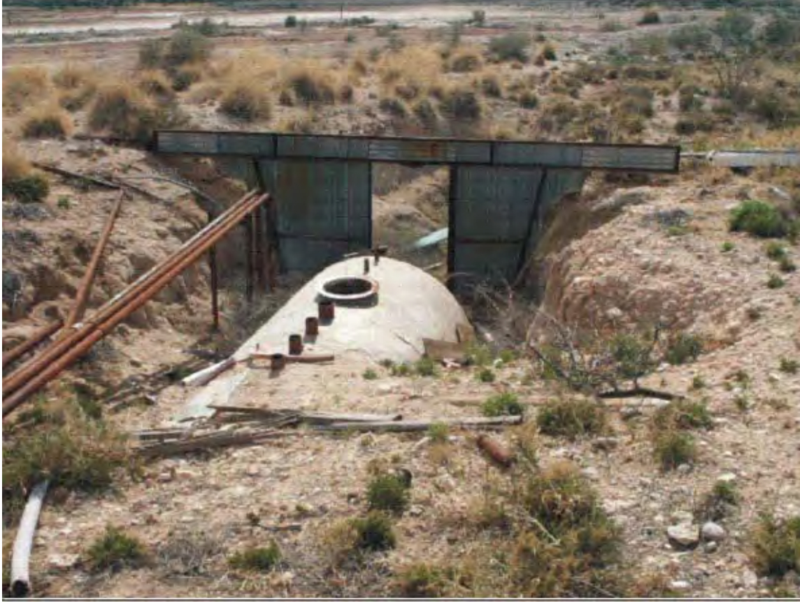
Figure 2.11.3-5 Plumbing and Partially Buried Tank at the Pollution Control Inc. Landfill Area
