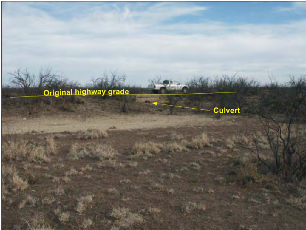
2.3.4.2-4 Onsite Drainage Culvert
