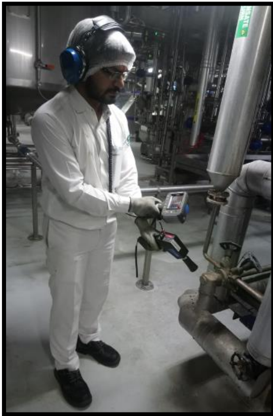
Steam Trap Monitoring
