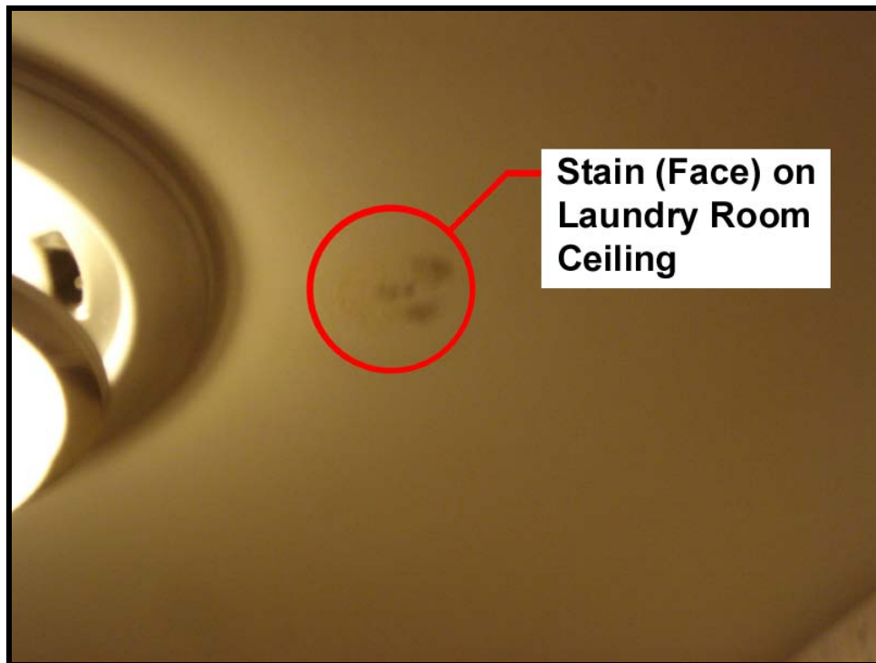
Laundry Room Ceiling – Image 6
