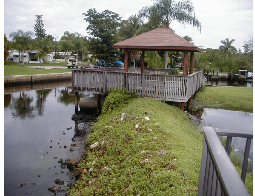
Community Stormwater Retrofits
