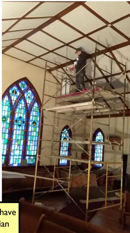
The light fixtures and the ceiling fans have been re-wired and hung. The electrician said there was evidence of a small fire in the attic around the wiring so we are lucky the church didn't burn down.
