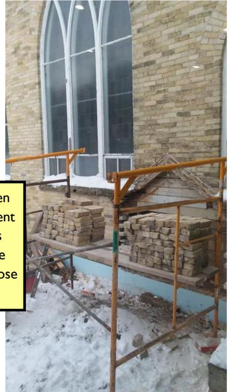
Brick work was done to fill in the open spaces where the door to the basement was previously located. Cornerstones has been put in place. Thanks to those who helped get the old mortar off those bricks; they were needed.
