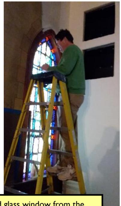
The newly exposed stained glass window from the pipe room. Bruce Bosben is working to strip old paint off the window frame.
