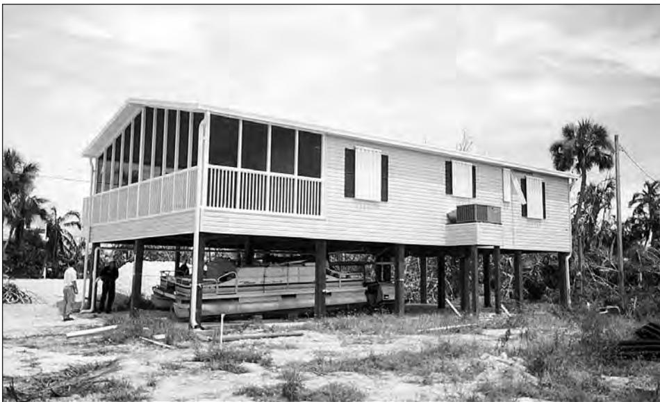
Figure 8-4. Manufactured home on a pile foundation.
