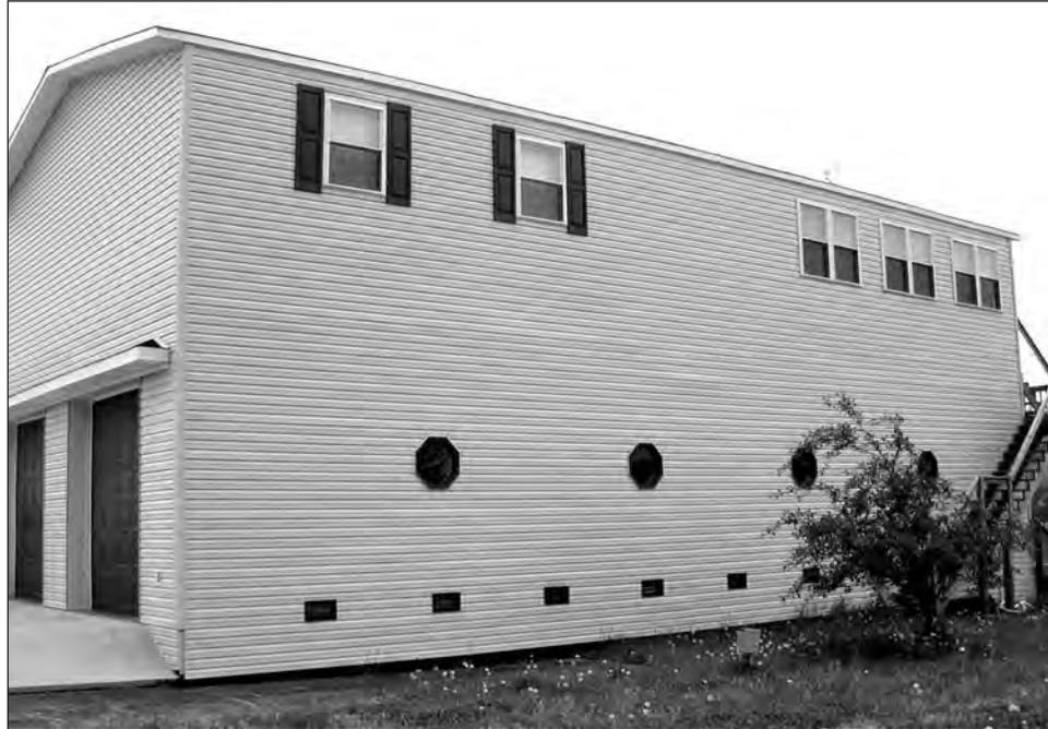
NFIP regulations permit enclosed foundations for manufactured homes in SFHA A zones with a requirement that the foundation walls include flood vents. 44 CFR 60.3(c)(5) requires that:
