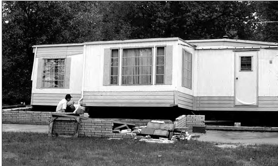
Figure 5-7. A manufactured home destroyed by the hydrodynamic forces of flooding.
