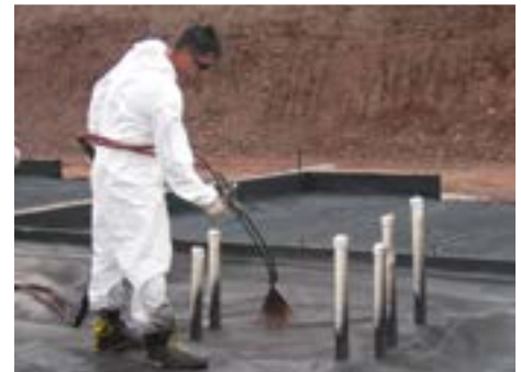
LIQUID BOOT® 500 spray-application effectively seals penetrations, footings, grade beams and other irregular surfaces that are considered critical vapor intrusion pathways.
