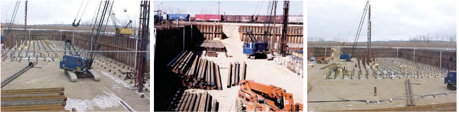
Pile were delivered from the mill by rail in lengths that had been determined by the pre-production pile-testing program.
