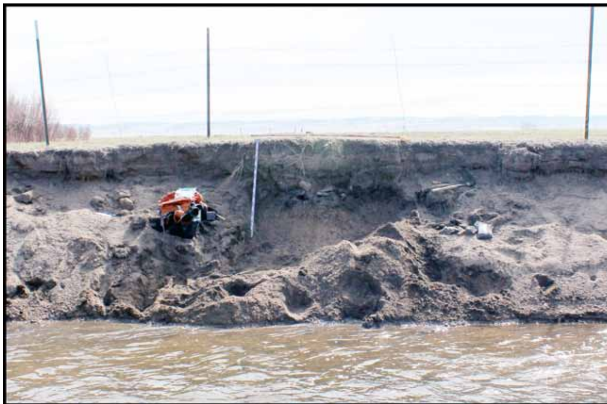
Figure 3: View of AB3354 facing east. Feature is visible in cutbank center near the tape.
