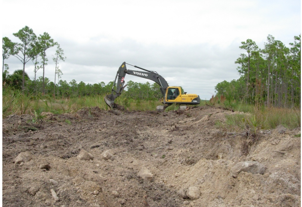
Removing berm and backfilling agricultural ditch
