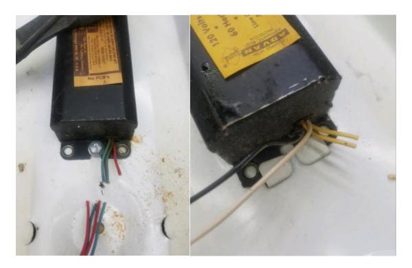
Connect the wires that fed the ballast (hot and neutral) to the wires going to the sockets. One to one end and one to the other. Wire-nut the connections and replace the cover.
