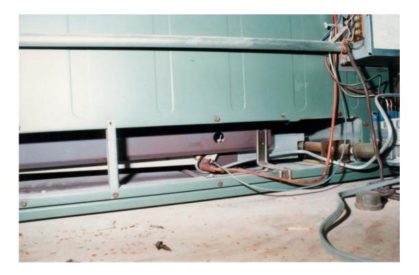
Photo Two: Combustion air intake port at bottom edge of furnace housing.
