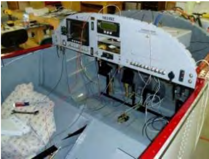
Panel with wiring in progress.
