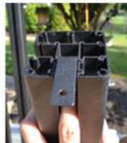
7) Slide bracket in post, use the inner slot. Short side down. Secure with a Hexagon screw .
