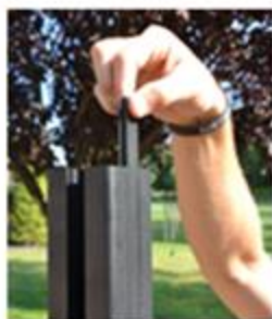
2) Remove channel covers from posts.
