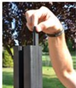
5) Remove channel covers from posts.
