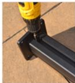
6) Slide bracket until it touches the base plate, secure with a hexagon screw .
