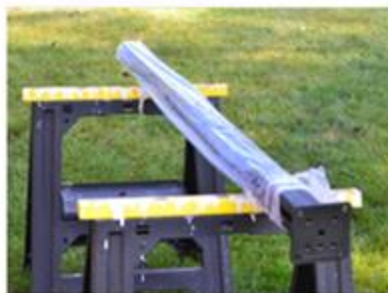
3) Tap in base plates into the bottom of the posts.
