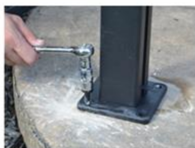
8) Adjust leveling knobs. Secure a 4 inch concrete anchor screw in each corner of the base plate.
