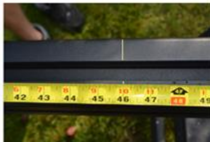
6) Measure down to 46 inches. Mark a pencil line. Top of bracket will be here.
