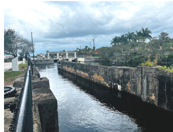
Looking west at the lock as it stands today.
