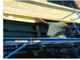
Vapor Barrier being installed over Dens Glass
