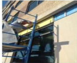
Dens Glass being applied over Hat Channel
