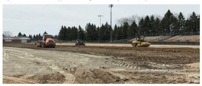
With the stabilization complete, the installation of the drain tile and stone base was able to move ahead. In addition, prep work for landscaping at the expanded drainage basin south of the Baseball Field has also started.
