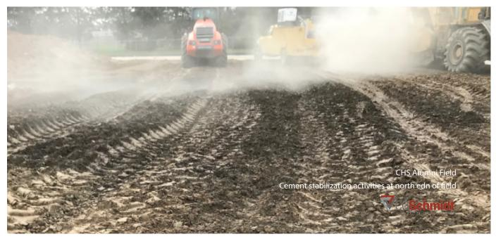
The warmer weather has brought renewed activities on the new Turf Field at Cedarburg High School. This month stabilization work, required to address spongy soils in the field area, was performed. This provided a very stable base needed to support the trucking and machinery used to complete the turf field installation.
