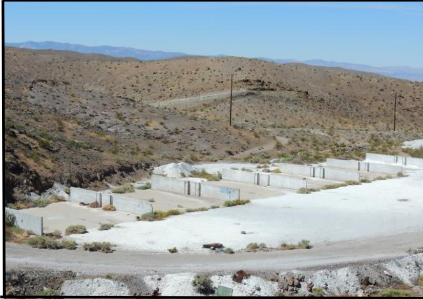
Loading Bins that were used to store different grades (purity) of Talc
