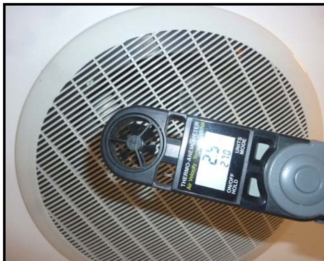
Figure 17 – Measuring air velocity.
