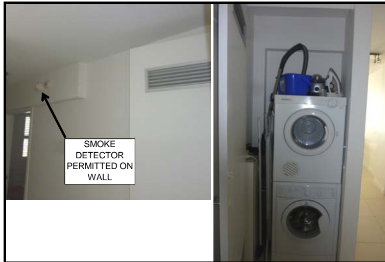
Figure 5 – Laundry with door top air grille
