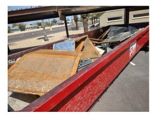
It was discovered the A/C ventilation system (ductwork) on the south side of the church collapsed! Clear Choice Mechanical, LLC has begun work to remove the collapsed ductwork and install replacement ductwork which will improve the efficiency of our air conditioners. With the new system, less cool air will be escaping in the coiffeurs of the church and be efficiently re-routed to cool the Sanctuary and Beehive. The project should be completed in time for the increase in summer temperatures!
