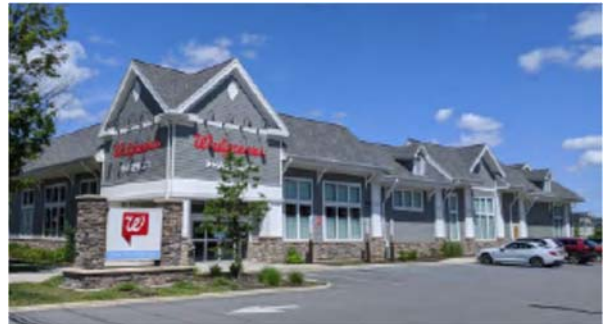
Figure 19. This is an example of a franchise business with building design elements and signage that incorporates many of the design standards desired for the TC District. Note rooflines, lighting, signage, bollards, side parking, side entrance and windows.
