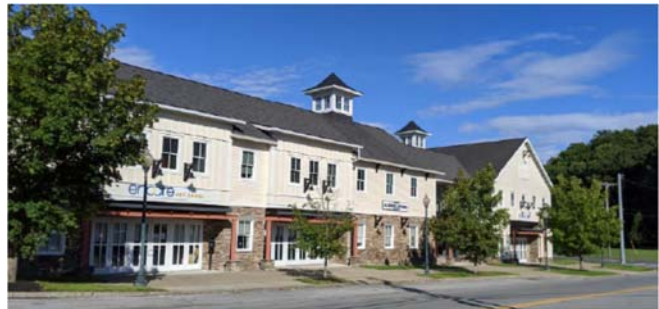
Figure 14. Example of a new building showing a roof design with cupolas consistent with the rural character in Union Vale. This also shows appropriate facade breaks used to improve the aesthetics of a large building.
