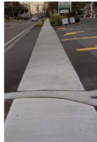
Figure 8. Example of a pedestrian sidewalk that continues through driveway to prioritize pedestrians.
