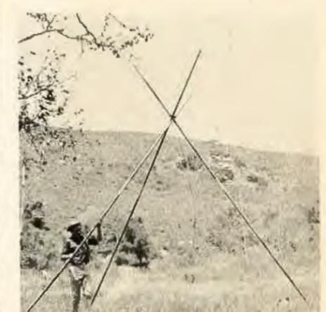
Two of the base poles are placed at their stakes and the third is used to lift them into the air.
