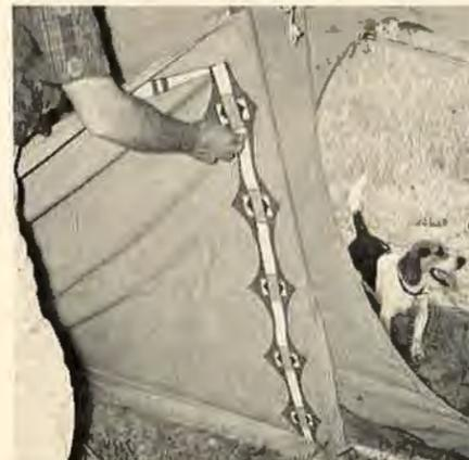
The liner on the inside is tied to a line strung around the poles. This creates an air conditioning by convection currents. To cool off you raise the height of the outer skin; to warm up your lower it.
