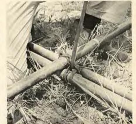
After the three bases are staked, the poles are removed and lashed together at the top with latigo leather straps.
