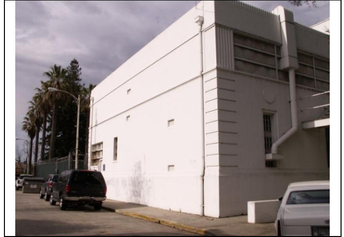
View looking southeast at the west elevation
