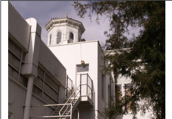
View looking northwest at the south elevation detail and cupola
