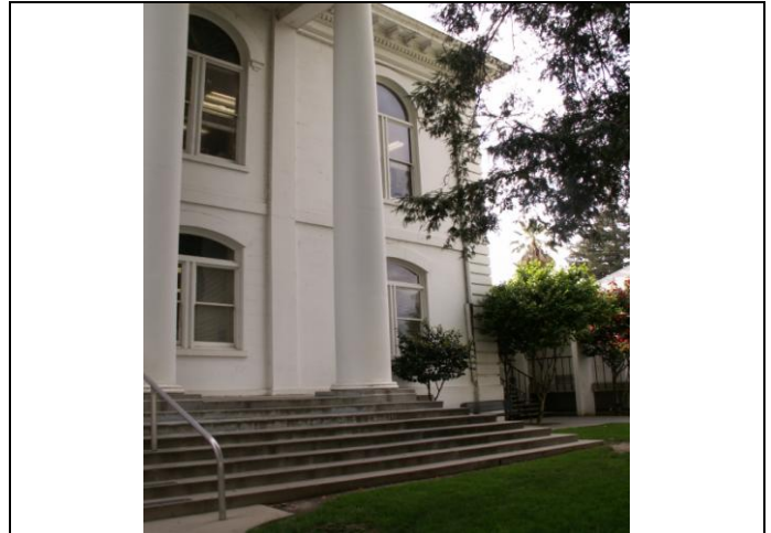
View looking southeast at the façade steps
