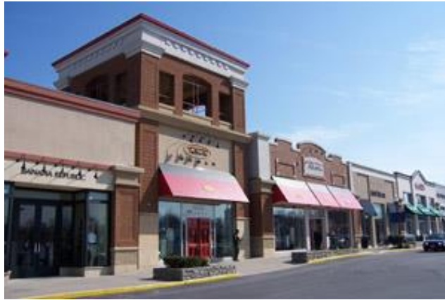
Figure 1210-E: Illustration of façade treatments such as pilasters, projections, and material changes to provide a visual façade offset. 12
