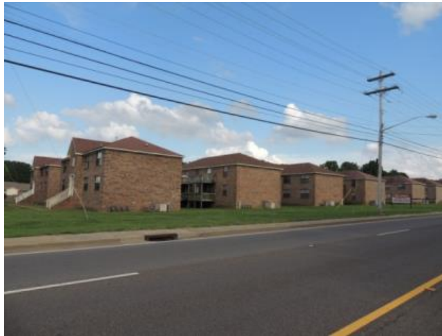
Figure 1210-C: Illustrative example of unacceptable architectural design for multi-family dwellings
