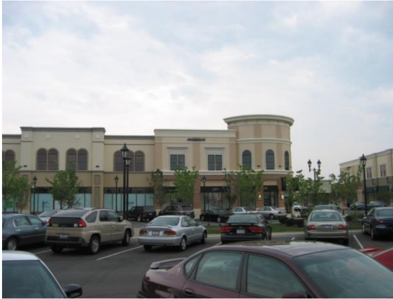
Figure 1210-F: Roofline changes shall be aligned with corresponding wall offsets and/or material or color changes.
