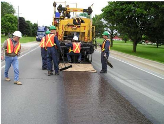
**Photo 13 – Micro-surfaced Joint**
