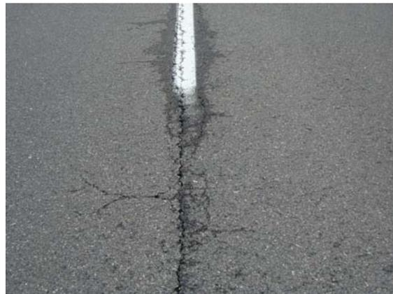
Photo 3 (below) shows an example of pavement deterioration originating at the joint between the left and right lanes.
