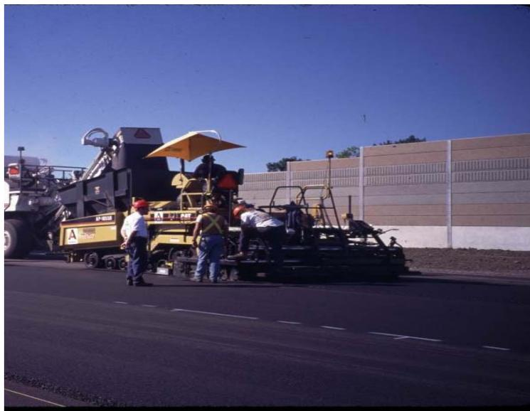
Equipment manufacturers have developed heaters (photo 6), compaction devices and adaptors for pavers to assist in compaction of the joint. While this new equipment can
