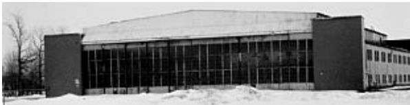
Former aircraft hangar
