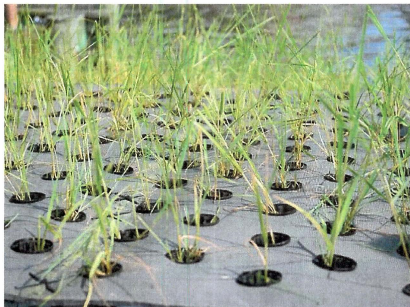
Volunteer residents of South Bethany Beach help install the floating wetland mats and plants that will be placed along the bulkheads in the South Bethany canals to help treat stormwater runoff on Tuesday, June 19, 2018. (Photo: Staff Photo by Megan Raymond)
