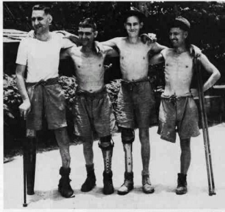
Australian survivors at Changi camp display artificial limbs of scrap metal and rubber, made by POWs' medics to replace legs that had turned gangrenous as a result of skin ulcers.
