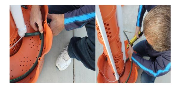
14. After you connect two of the hoses you are ready to complete the circle by connecting the hose from the AquaJet to the tee of the hose that comes in from the outside. See below.
