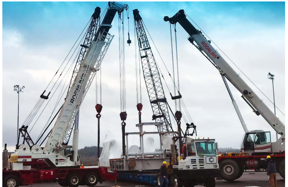
Local contractor Rognlin's, Inc. used four cranes to lift a record heavy piece of over-high, over-wide equipment at Terminal 4 last month.
