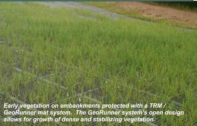
Early vegetation on embankments protected with a TRM / GeoRunner mat system. The GeoRunner system's open design allows for growth of dense and stabilizing vegetation.
