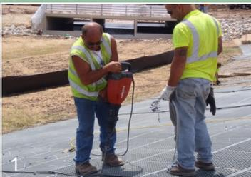
Photo 1. A pneumatic driver speeds the driving of anchors; reduces worker fatigue.
