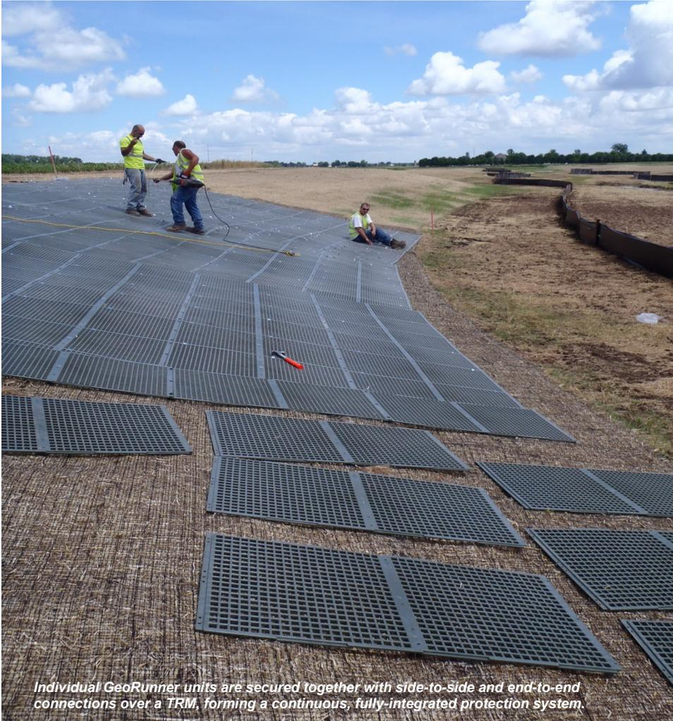
Individual GeoRunner units are secured together with side-to-side and end-to-end connections over a TRM, forming a continuous, fully-integrated protection system.
