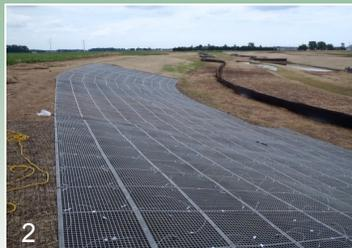
Photo 2. Completed GeoRunner embankment prior to trimming of anchor wires & vegetation growth.
