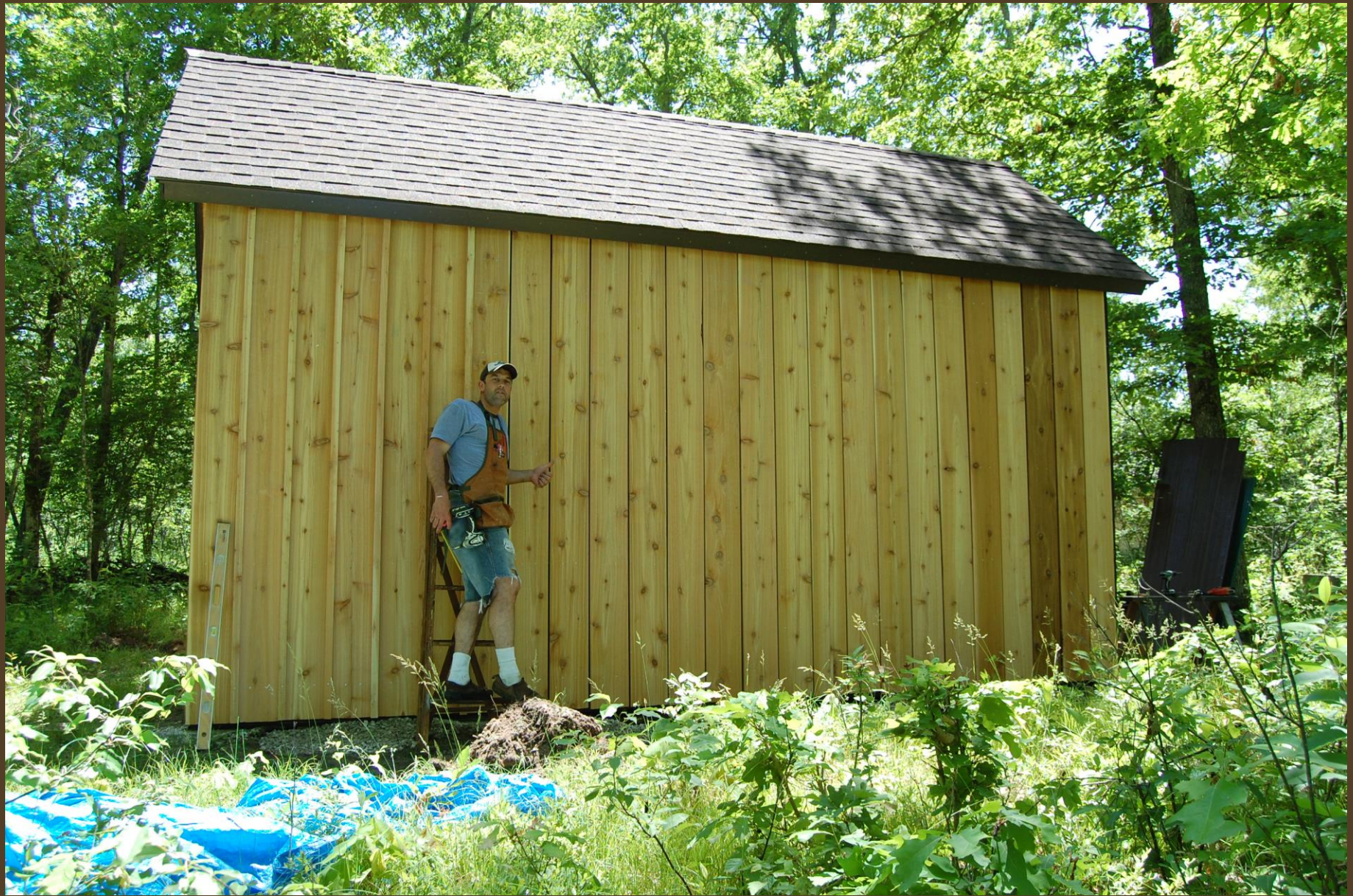
North wall almost done...just the battens left.
