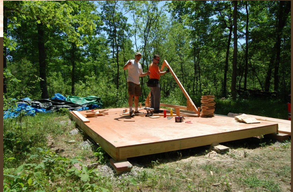
06/09/12: Mike Endres joined me for this next phase...the truss build!
