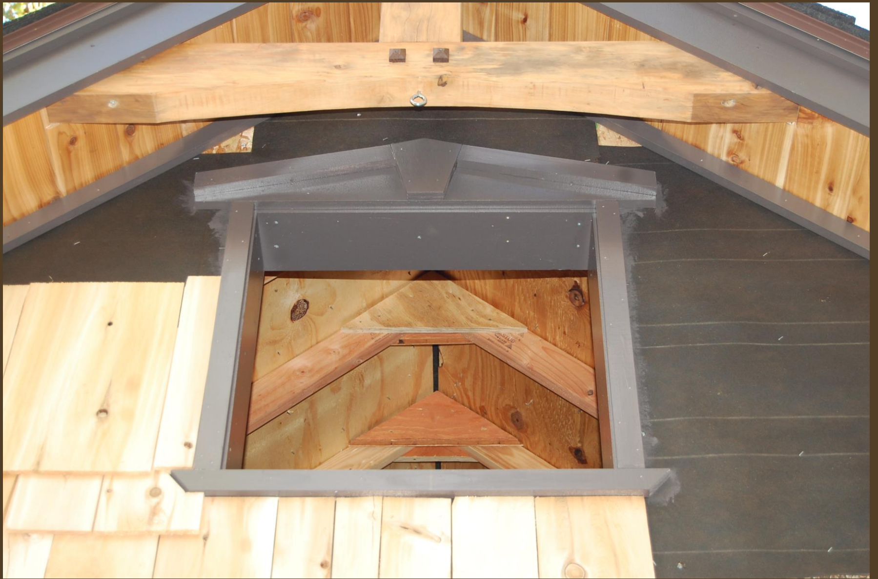
Here is the loft door with the finished framing.
