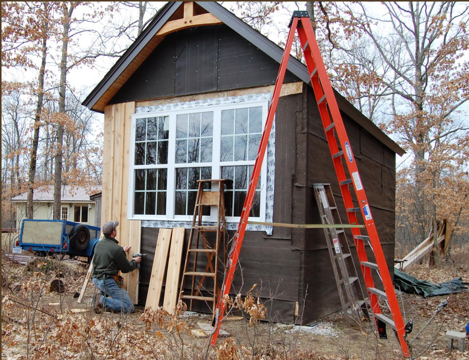
Next the fun part! Installing 1x8 cedar board siding.
