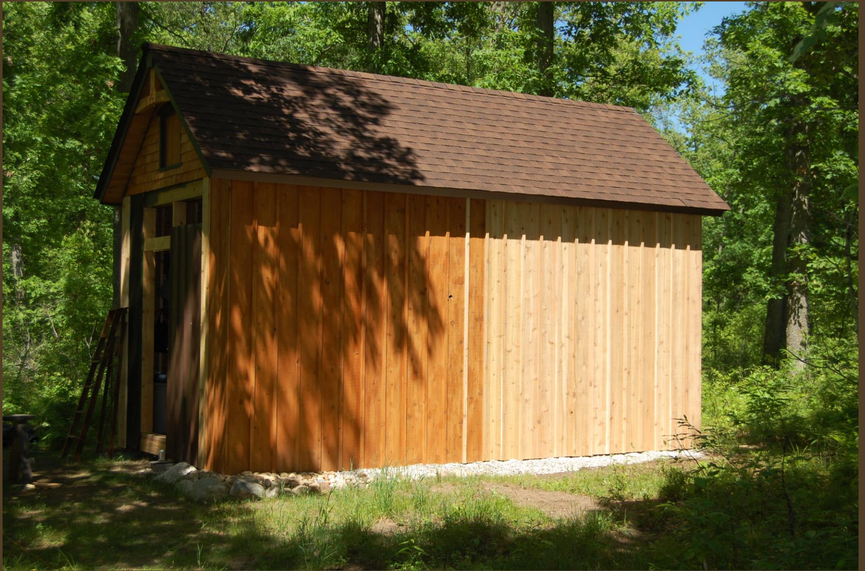
South wall exterior complete...just need to stain the new boards.
