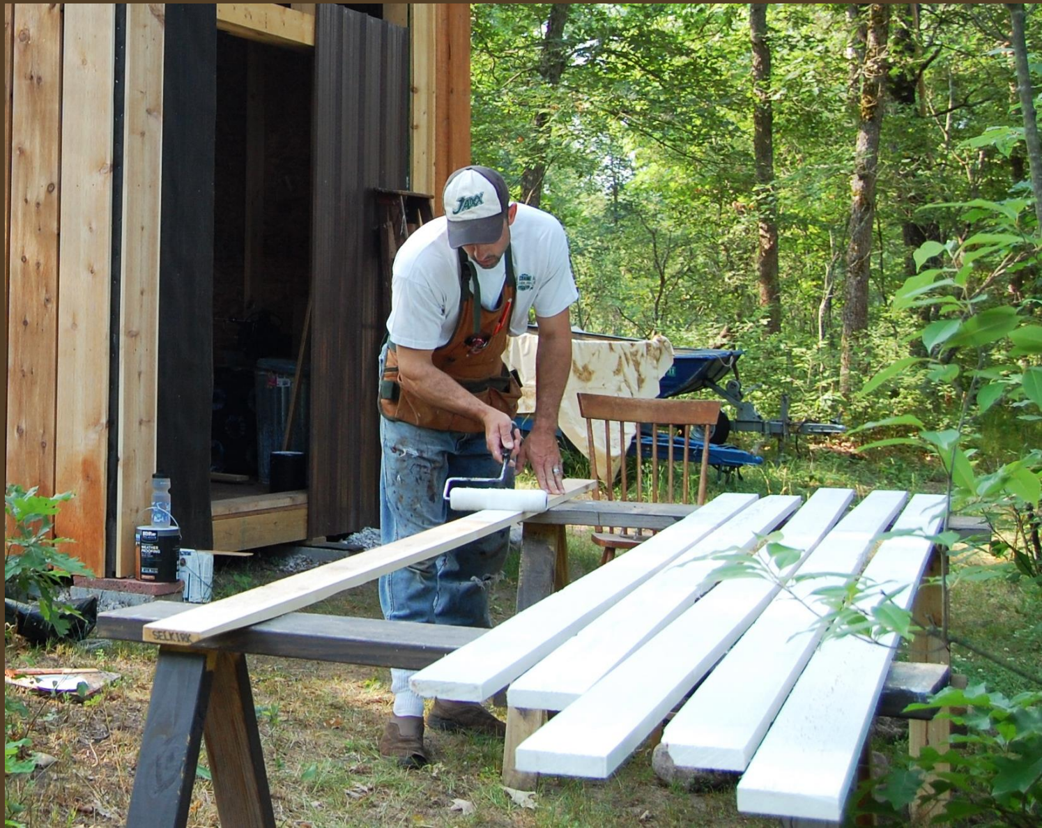
Prepping the trim boards with a coat of primer.
