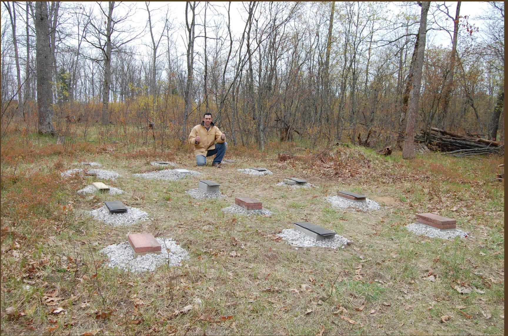
04/29/12: Back up here again...finished leveling the foundation footers.
