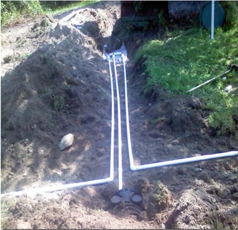
Manifold with three lateral connections.
