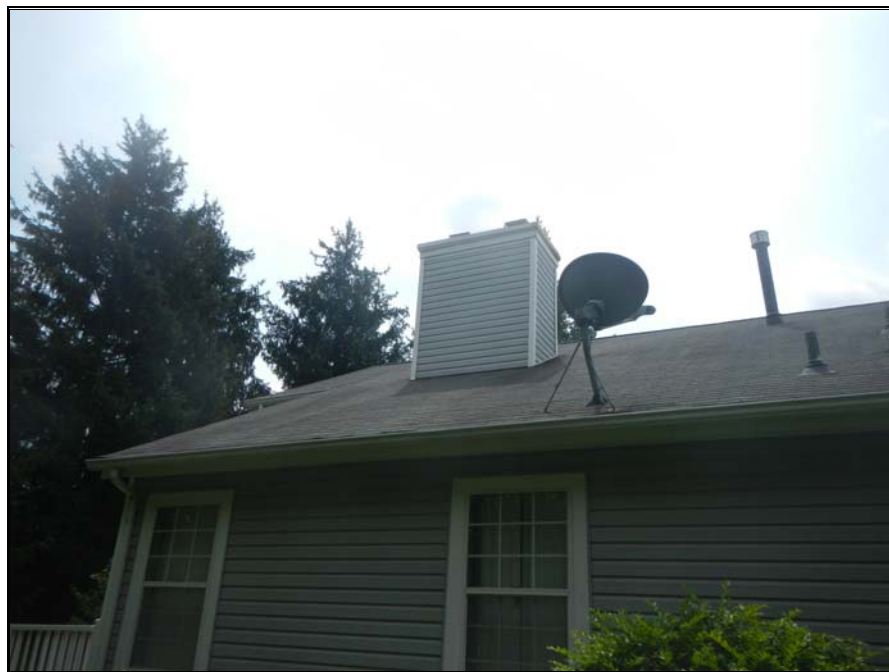
Photograph 20: Typical view of roof shingles and chimney chase cover/cap
