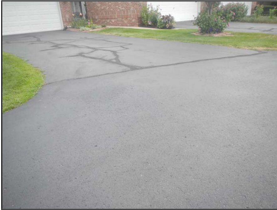
Photograph 25: Typical view of asphalt driveway
