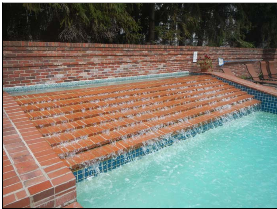
Photograph 10: Typical view of pool waterfall feature
