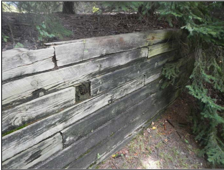
Photograph 18: Typical view of wood retaining wall
