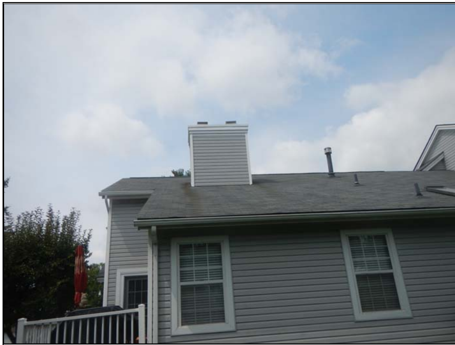
Photograph 22: Typical view of roof shingles
