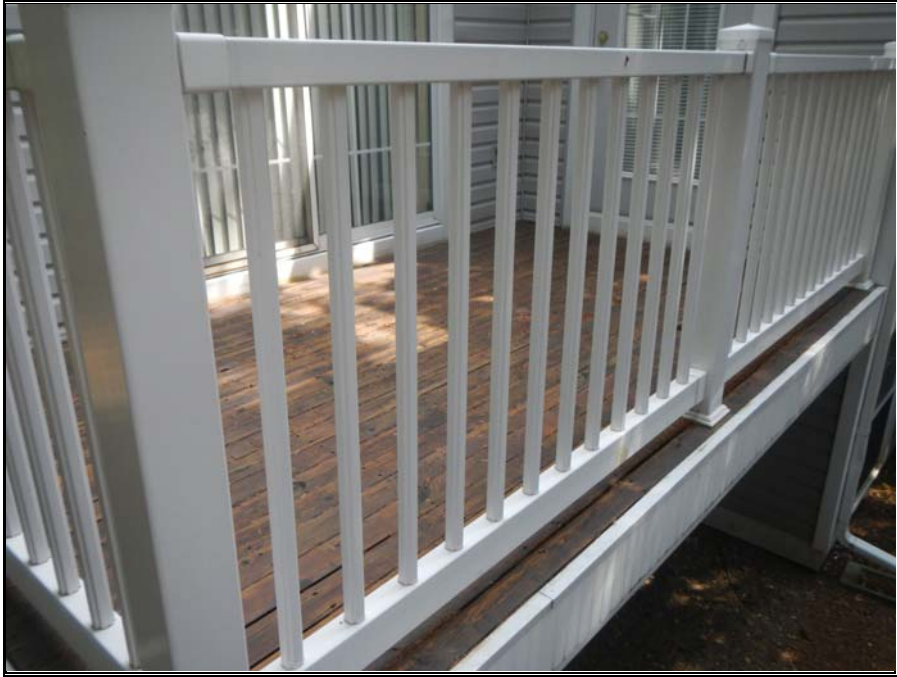
Photograph 14: Typical view of wood deck
