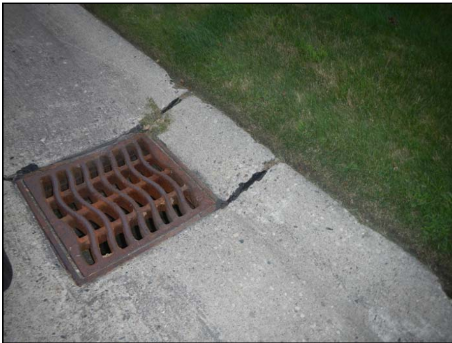
Photograph 24: Typical view of catchment basin
