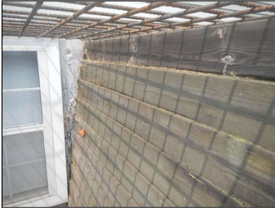
Photograph 21: Typical view of window well wood retaining wall
