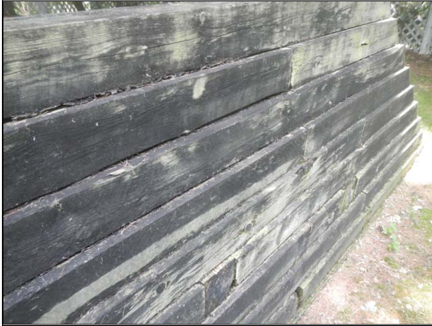
Photograph 15: Typical view of wood retaining wall
