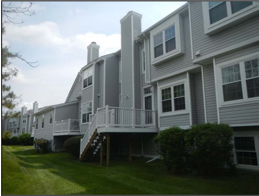
Photograph 17: Typical view of exterior building elevation
