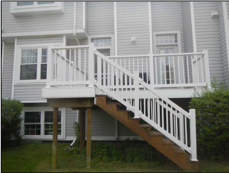
Photograph 16: Typical view of exterior building elevation
