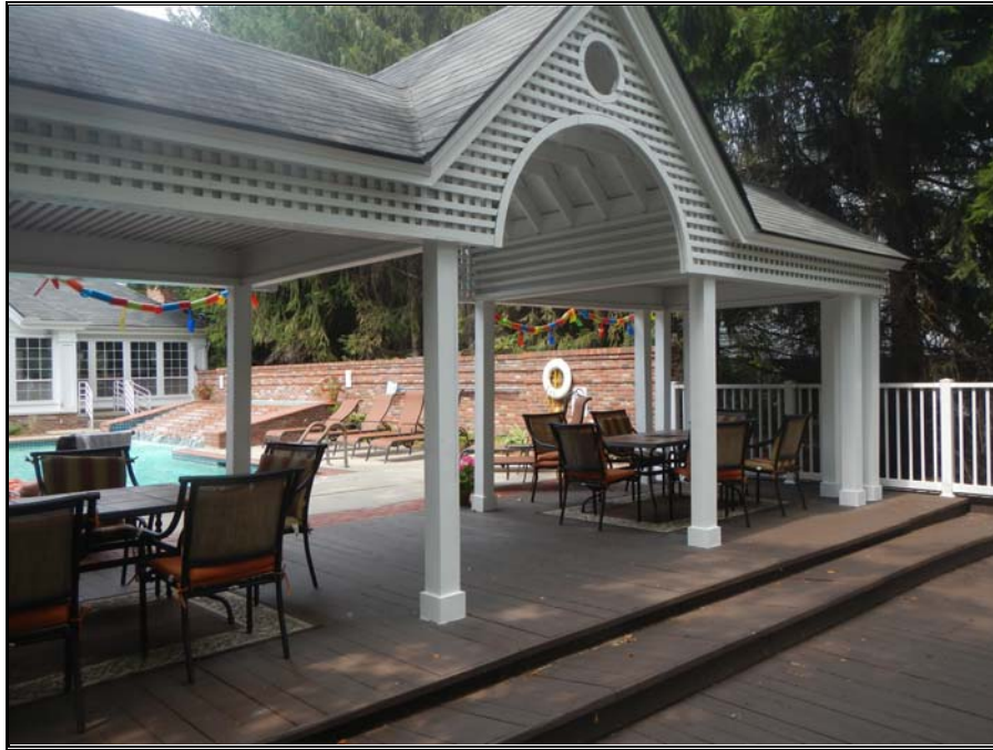
Photograph 9: Typical view of gazebo area
