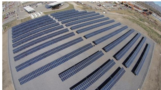
Salt Lake City completed a 1 MW solar photovoltaic farm on a former landfill site at 1955 West 500 South in 2014. Existing incentives for solar, including a 30% federal tax credit which expires in 2016, can reduce the upfront expense of installing panels. DPU has the opportunity to install a solar farm more than three times the size of the landfill solar farm at the Terminal and Park Reservoirs.
