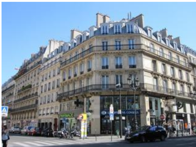
Beautiful buildings along Rue du Pont Neuf and Rue de Rivoli
