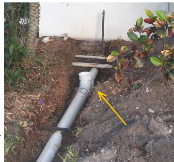
Required by code: New 4 inch cleanout installed near the house.
