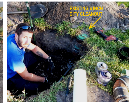
Fittings being installed at the connection to the city system.
