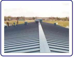
The subject facility is a functioning elementary school that was originally constructed in 1970 based on the "open-campus" concept with independent building enclosures tied together with open air covered walkways. The existing roof was a gravelsurfaced built-up roof membrane over a lightweight insulating concrete fill and metal form deck supported by open-web steel bar joists. The slopes of the roofs ranged from 1/4-inch to 1/2inch per foot to 2-inches per foot.
