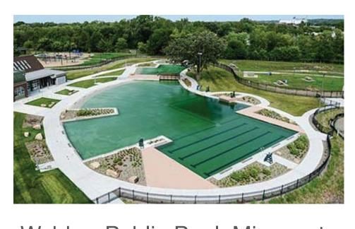
Webber Public Pool, Minnesota: This public pool is a completely natural pool. With lap lanes, zero entry, and deep end with diving area this poop is naturally filtrated with plants and microbes and has a 16,250 s.f. regeneration basin.
