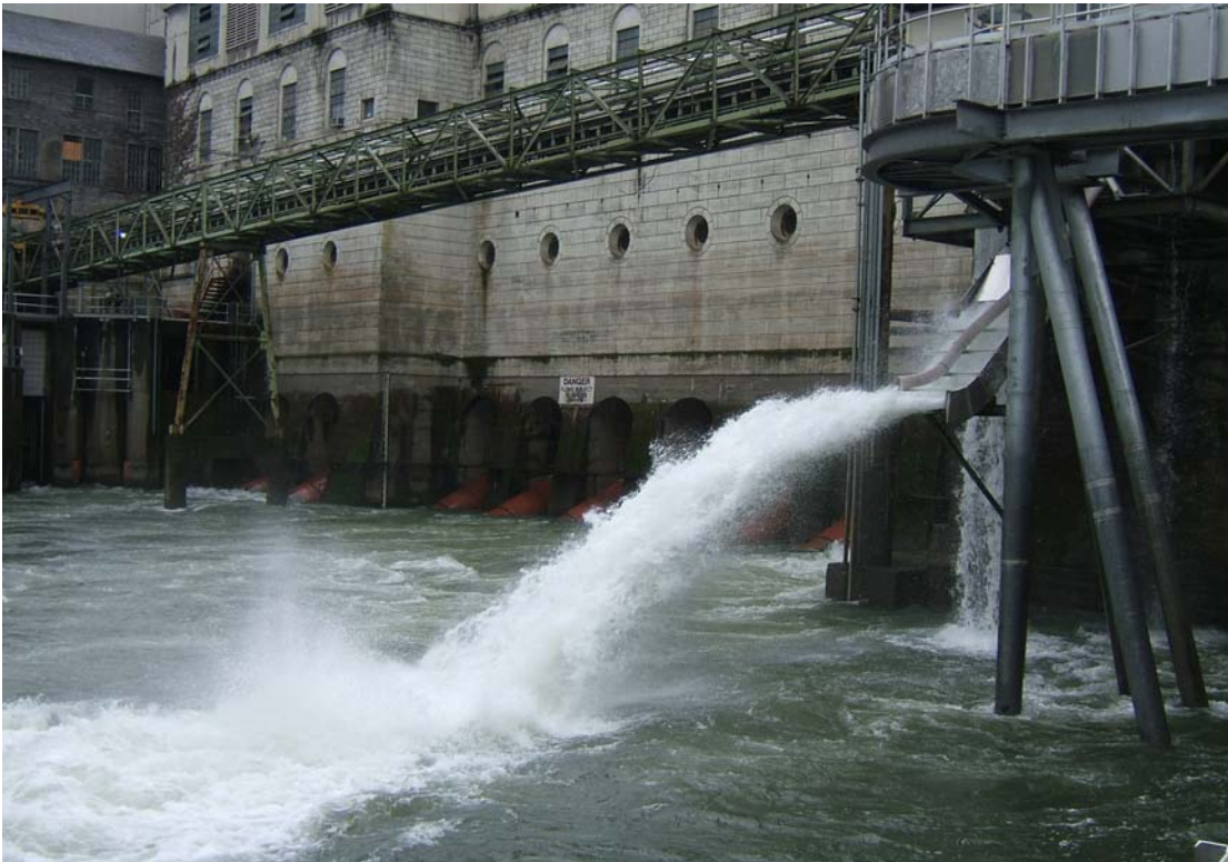
Figure 10. Unit 13 Outfall Chute operating at approximately 30 cfs.
