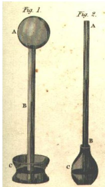
On the Left, A Galileo Thermoscope (thermometer)
