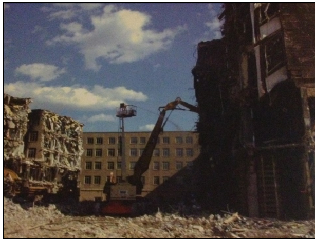
ABOVE: The Pentagon in Arlington County, Va, after the attacks on Sept. 11, 2001. Five floors of three separate buildings — a fifth-mile long, comprising office space, hallways, and restrooms — required total reconstruction.
