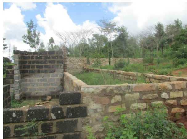
Kavonge church building expansion
