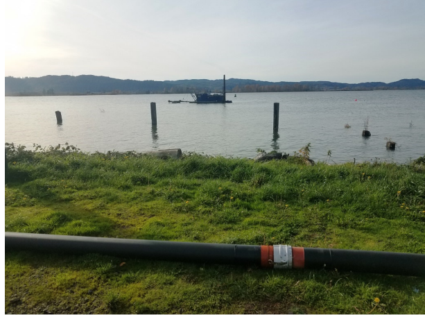
Dredge and spoils hose
