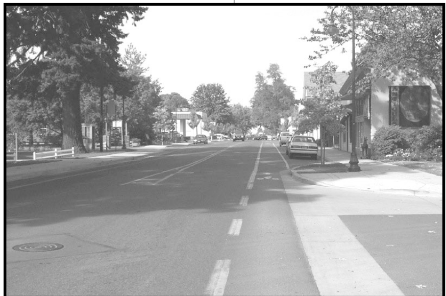
Newly installed sidewalks and bike lanes in downtown Coburg.
