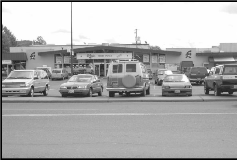
Commercial parking to the east of the railroad is accommodated entirely through private parking lots.
