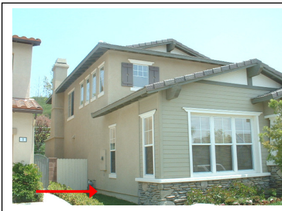
Proper clearance from Weep Screed at left side of house.
